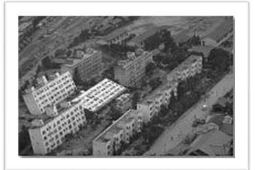
When liquefaction occurs, the strength of the soil decreases and, the ability of a soil deposit to support foundations for buildings is reduced as seen in the photo (SC) of the overturned apartment complex buildings in Niigata in 1964.
