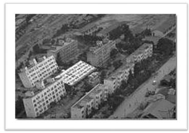
When liquefaction occurs, the strength of the soil decreases and, the ability of a soil deposit to support foundations for buildings is reduced as seen in the photo (SC) of the overturned apartment complex buildings in Niigata in 1964.
